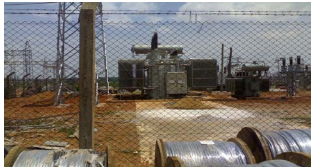
Transformation Substation under construction
