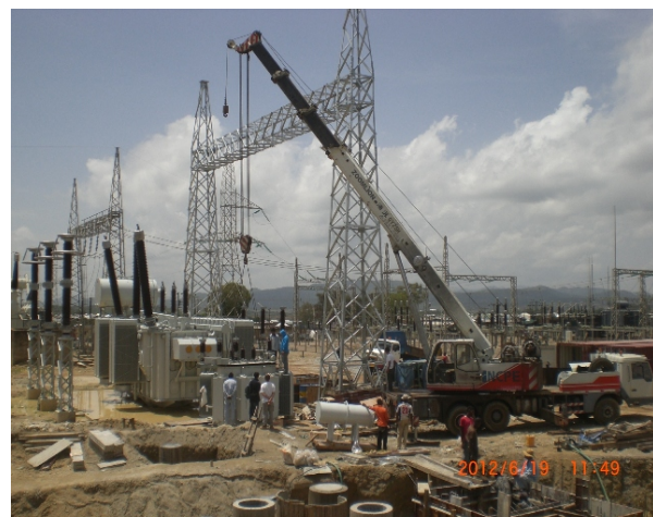
Earthing transformer installation operation for Jos S/S
