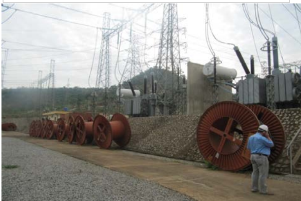
150 MVA 330/132/33 Kv Transformer reinforcement at Katampe, Abuja – Completed and Commissioned
