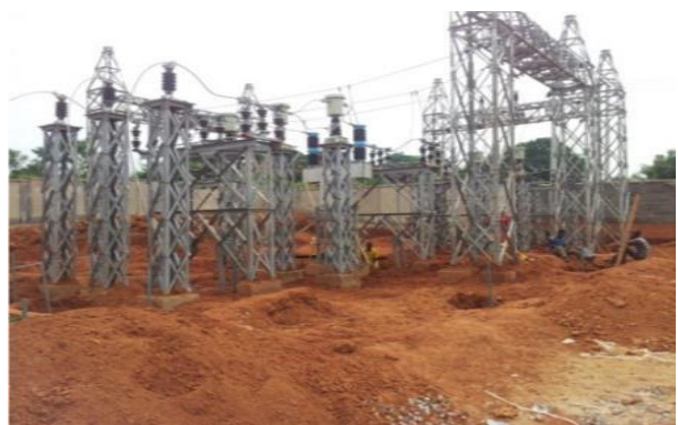
Gantry Structures Under Construction
