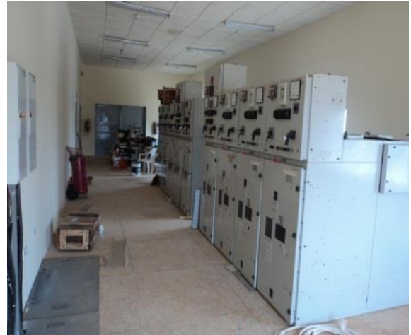
Completed - Installation of substation indoor panels
