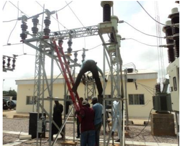
Pre-commissioning Exercises in Progress
