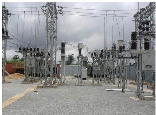
Works at Advanced Stages at an Injection Substation
