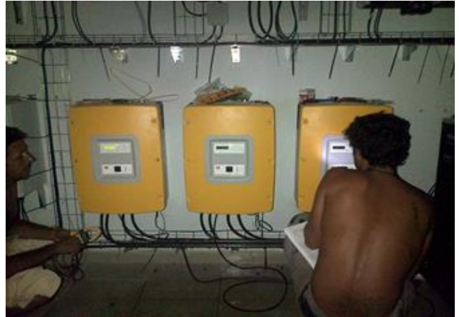
Cable termination in the control room.
