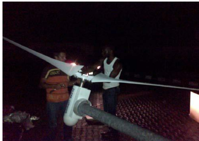
Installation of the wind turbine generators and blades.
