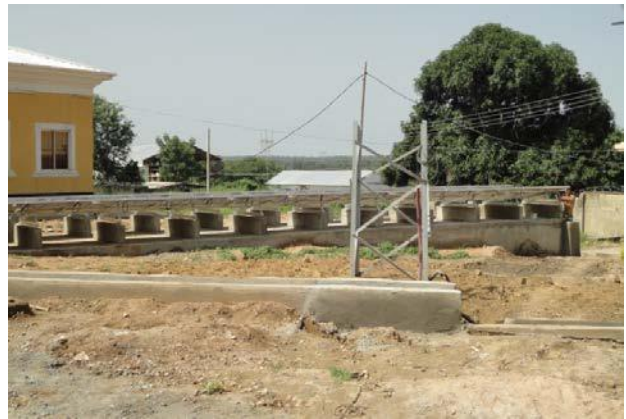
Connected Solar panels arrays installed on the site.
