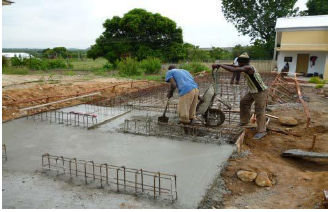
Construction of Solar Modules Foundation
