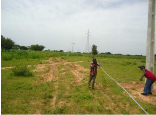
Stringing of the overhead line in progress
