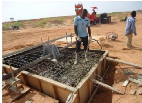
Casting of foundations
