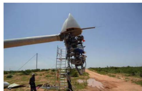
Nacelle installation
