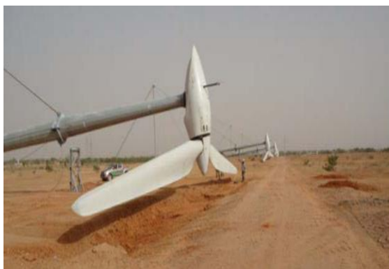
Uncommissioned 2 blade rotor Vergnet WTG
