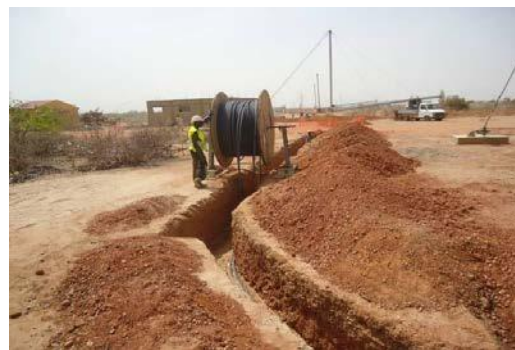
Internal Fibre optics in the Windfarm
