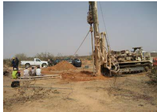
Drilling of micropiles
