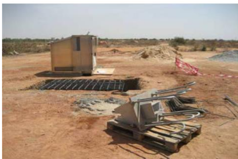
Electrical shelter installation
