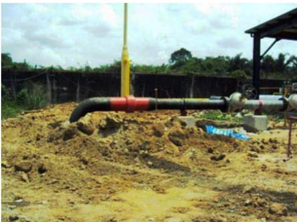
Sapele: Gas Pipeline tie-in to the Power Plant Receiving Station
