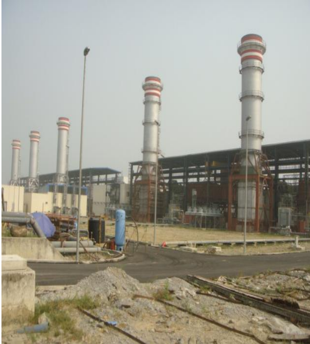
GTG Power Plant at Calabar LOT 1 - 562.5 MW
