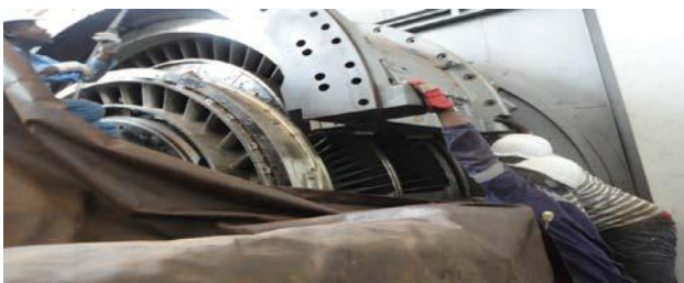
Inspection of Turbine Casing in Progress
