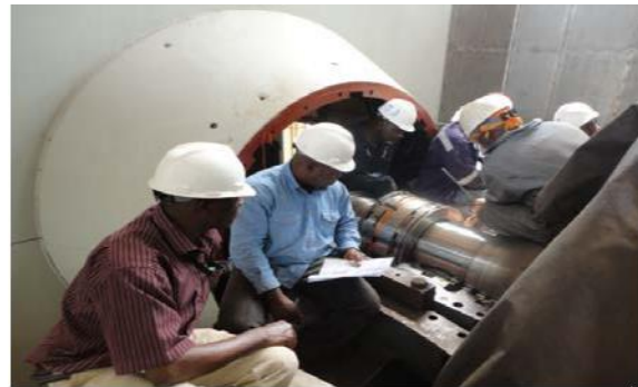
Major Inspection at Ihovbor Power Station
